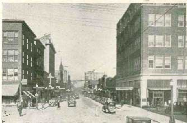
Street Scene 11th Street and Phillips Avenue
